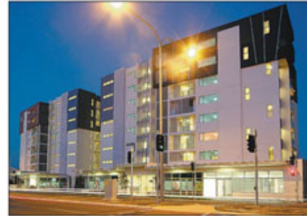
The Wharf complex at Robina is set to house a Metricon Homes tile studio
