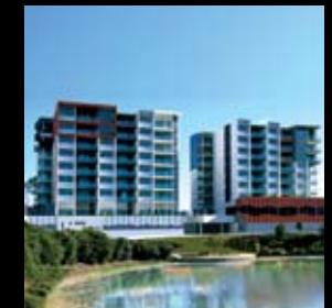
+THE WHARF 2009. Located adjacent to The Rocket, The Wharf is a twin 8 storey mixed use development of apartments and business space.
